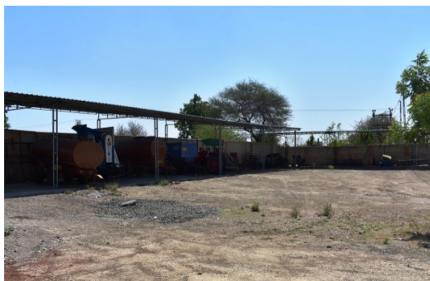
FARM IMPLEMENTS SHED
